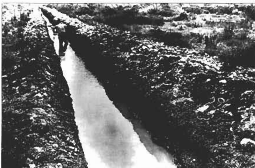
Fig. 3 - Drain being excavated by hand in South East karst district c. 1947. Photograph by South East Drainage Board, S.A.)
